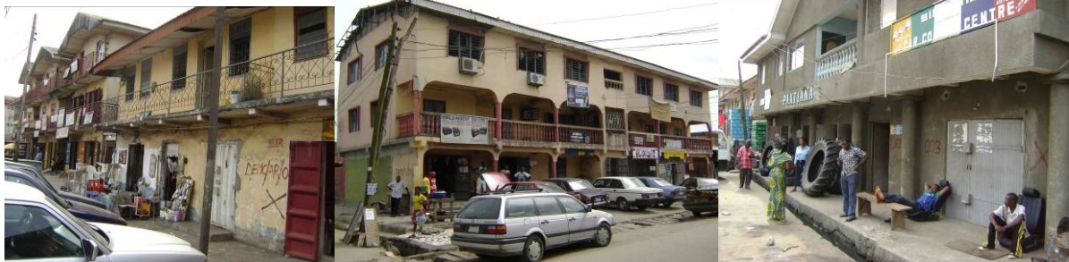
Legal buildings containing numerous rental units on Azikiwe and Ojoto streets, marked for demolition
